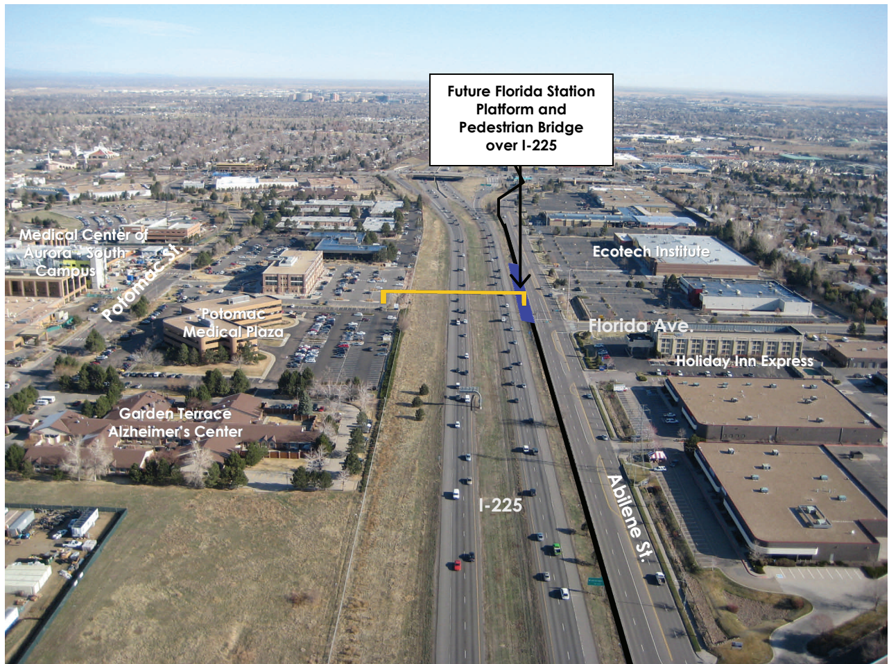
Figure 1. Aerial view looking north along I-225 and over the Florida station area
